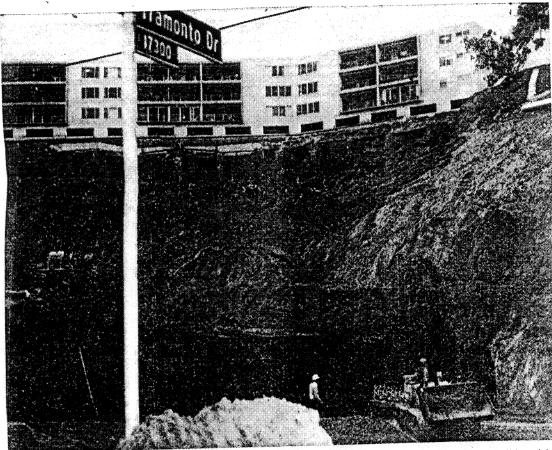
SPENDING \$279,000 funded for remedial grading work by Ocean Woods Terrace condominium (background). workmen remove existing unstable fill and replace void with sandy soil on Tramonto Drive's dedicated and undedicated roadway, northerly slopes of landslide-strick en structure and other hillside properties south of inter section with Los Liones Canyon Drive. Combined repair bill is expected to total \$561,000. -Palisadian Post Pho
